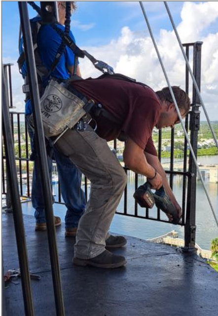
Cutting away the old railings.
