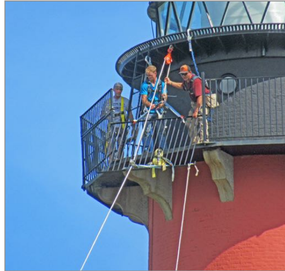
Hoisting a section of new railing.
