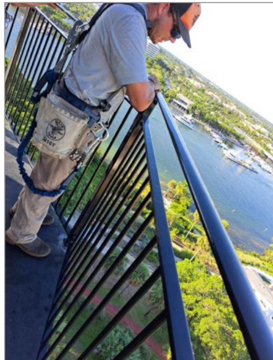
The completed railings
