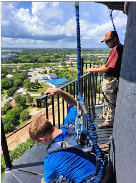
Installing the new railings
