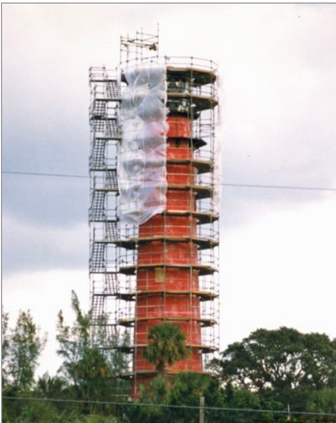
Jupiter Inlet Lighthouse undergoing major restoration 1999-2000
