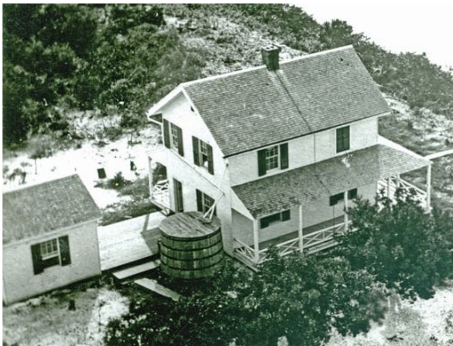
The 1883 Head Keeper's Dwelling viewed from the Lighthouse. The in-ground cistern was located under the wooden breezeway connecting the house and kitchen. The roof gutters can be seen leading into the large barrel cistern that provided additional water storage.
