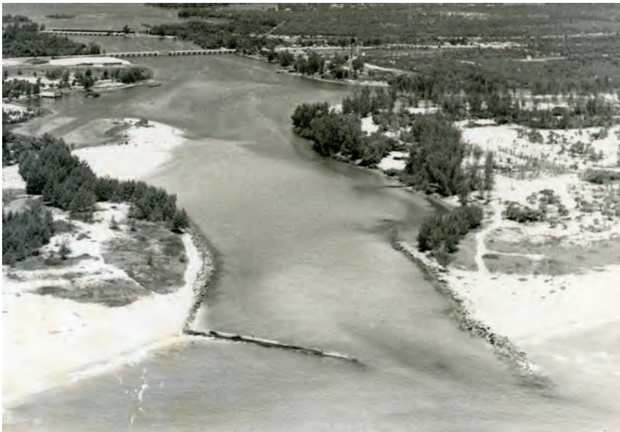
Jupiter Inlet circa 1953. The angular groin was added to the south jetty as part of reopening the inlet to navigation after World War II.
